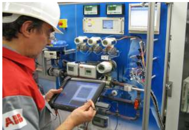
Fig. 1 Measurements: mobile device and WSN at industrial test-rig
